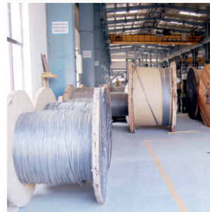
Underground Cable Laying (Power: 220 kV)
