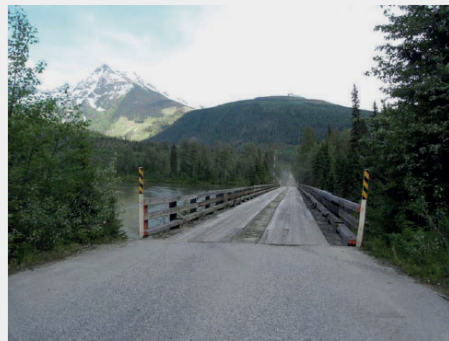
Access to site via bridge across the North Thompson River, immediately east of major highway
